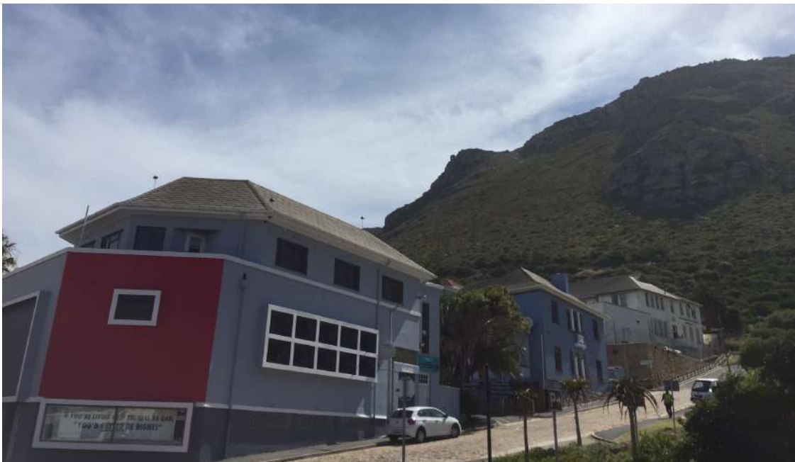
The CCFM Lecture Hall, with a new coat of paint in 2019.
